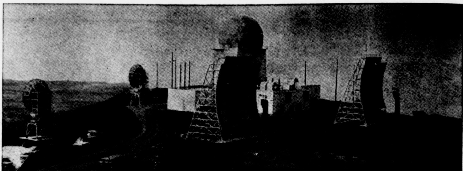
OUT OF THIS WORLD—Other-worldly look of the structures, above, fit the bleak site on which they're located. On Unimak Island, far out in the Aleutian chain, the group of buildings are part of the westernmost link of the transcontinental DEW—Distant Early Warning—network. Churchlike dome, center, houses radar unit. "Dishes," left, and curved reflectors, right, are portions of radar detection and beam-casting communications equipment.
