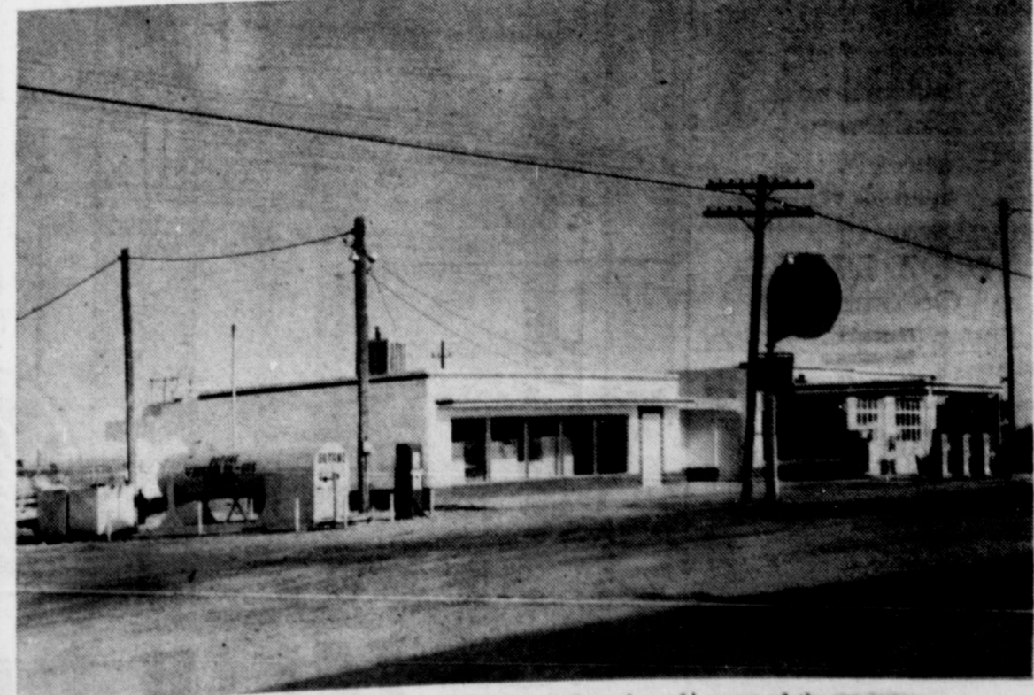
ANNIVERSARY — Vaughan Oil and Gas Co., at 1015 North Main, Winters, will hold their 25th anniversary Friday and Saturday of this week. Shown is the main service station and appliance show rooms of the company. (Photo by Little)
