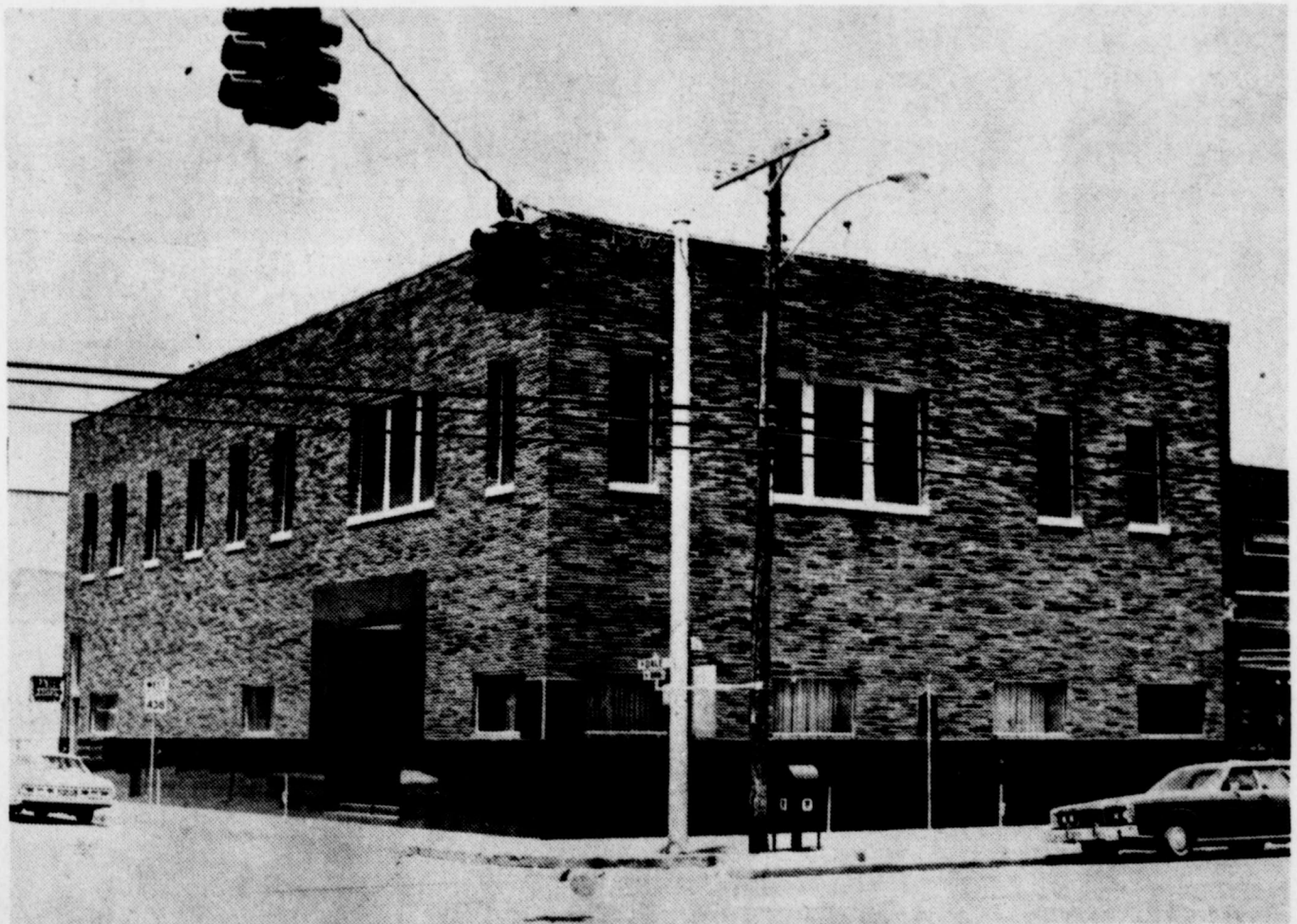
BANK BUILDING JUNE 7, 1975
