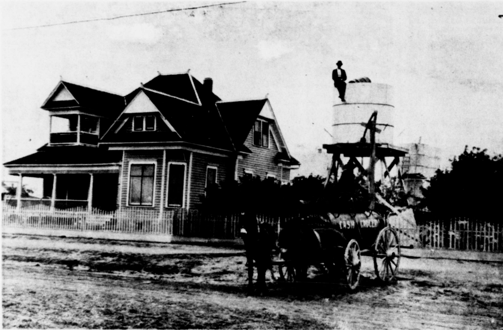
LEE BEDFORD WELLS - source for the first running water for the fast-growing City of Winters, in the early 1900s. The wells were abandoned many years ago, but there still are some who remember returning to these wells during some of the dry years, when lake water was not sufficient to supply the needs of the town.
