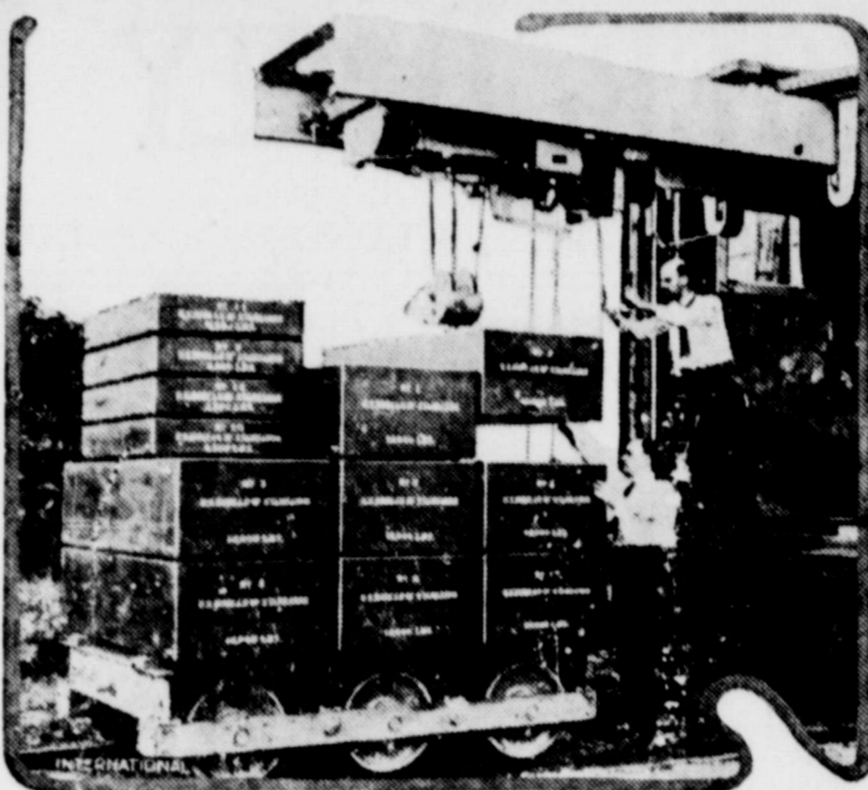
A railroad track scale testing car of the national bureau of standards, Washington. The car is fitted with weights of 10,000 pounds each, and is sent about the country to test railroad track scales. It also sets the standard by which is calibrated the test cars of the railroad companies.
