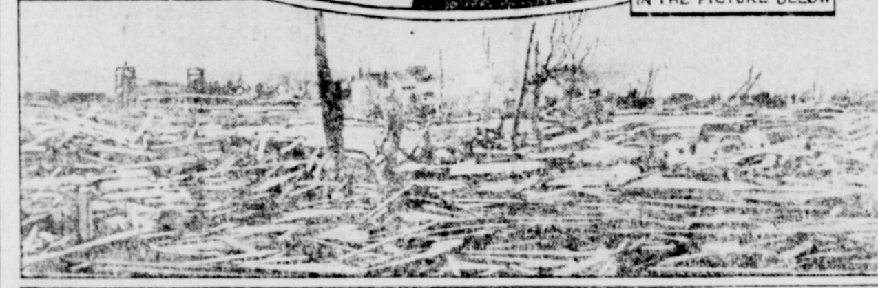
SWEEPED CLEAN FROM END TO END, GRIFFIN, INDIANA, A FEW HOURS AFTER THE GREAT TORNADO OF MARCH 18, 1925.
