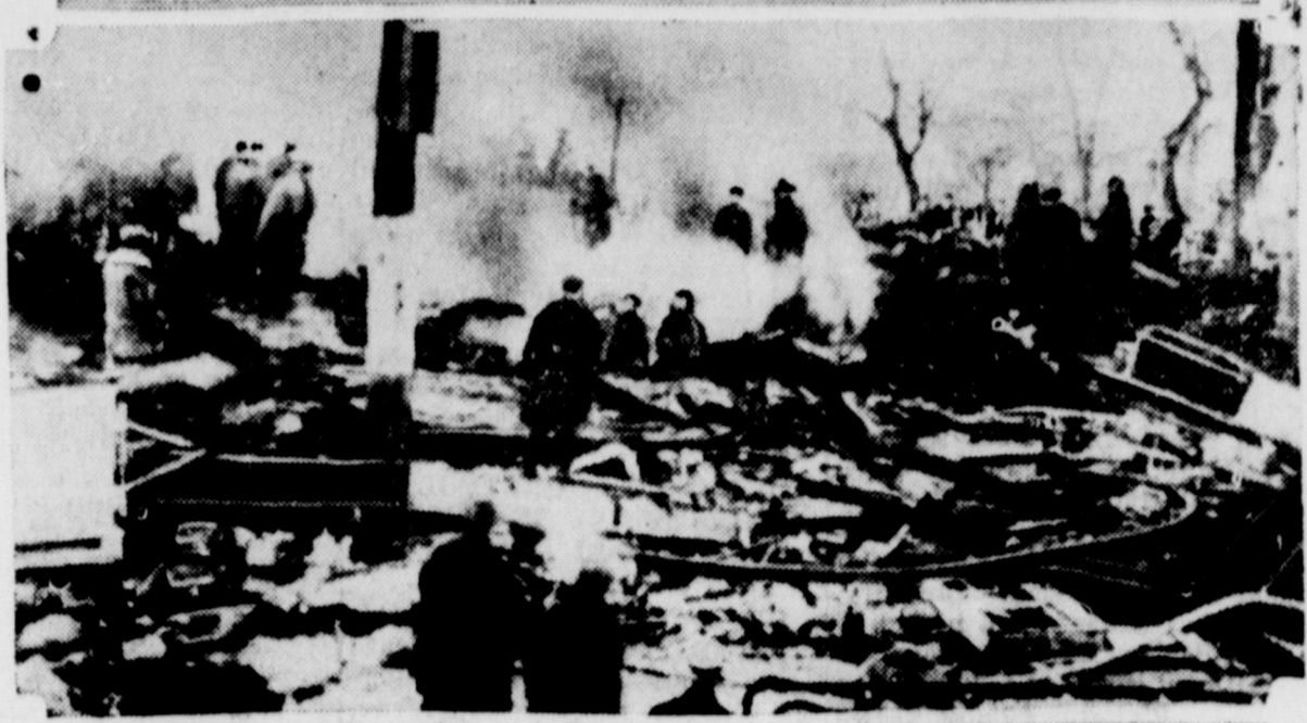
Here is a general view of the building at Newton, Mass., that was totally destroyed by a terrific blast caused by the explosion of a liquor still on the prem- ises. Seven people were killed in the explosion and subsequent wreckage of the structure. (International News)
