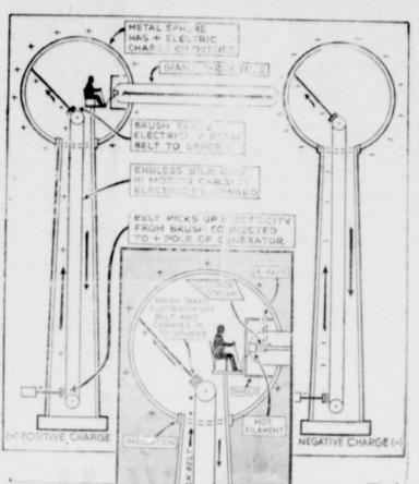
A machine to develop 20,000,000 volts of electricity, the greatest power ever produced by man, is to be constructed at the Massachusetts institute of Technology. The power will be developed by means of two spheres 15 feet in diameter. Dia-
