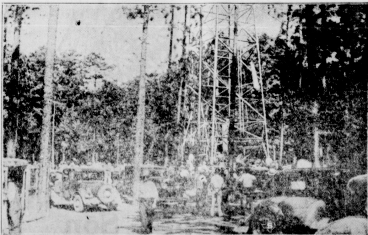
Here is a new oil well which definitely opens an entirely new field at the edge of the Big Thicket at Hook's Switch, Hardin county, 18 miles north of Beaumont. It is the Republic Production company and Houston Oil company's Ariola No. 1. The well is producing 5000 barrels daily of 40 gravity oil from a depth of around 4000 feet. Two other wells are already being drilled in the area. Five major oil companies are leasing land in the vicinity.
