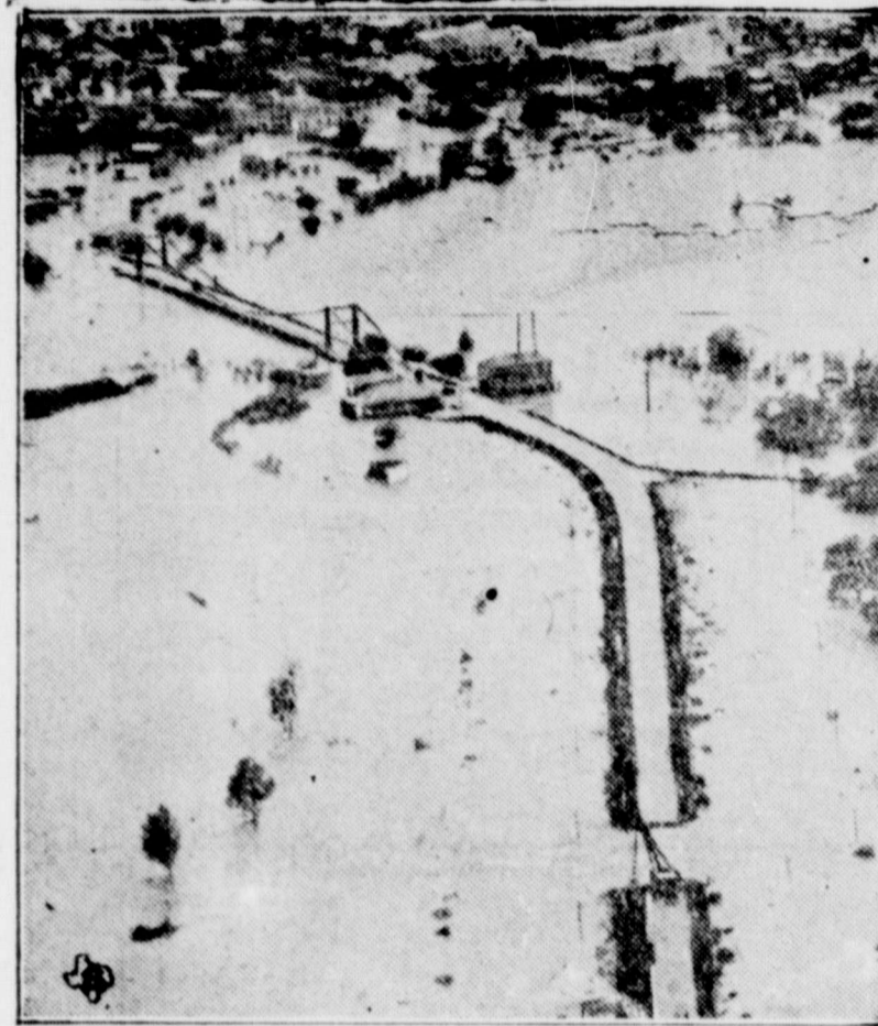
The extent to which the raging Rio Grande surged through lower valley lowlands is clearly shown in this excellent air photo. The international bridge from Hidalgo, Texas, to Reynosa, Mexico, is shown, the approach on the Mexican side inundated, while the furious water cut a 150 channel through the road on the American side. Hidalgo was isolated by the water for 50 hours.
