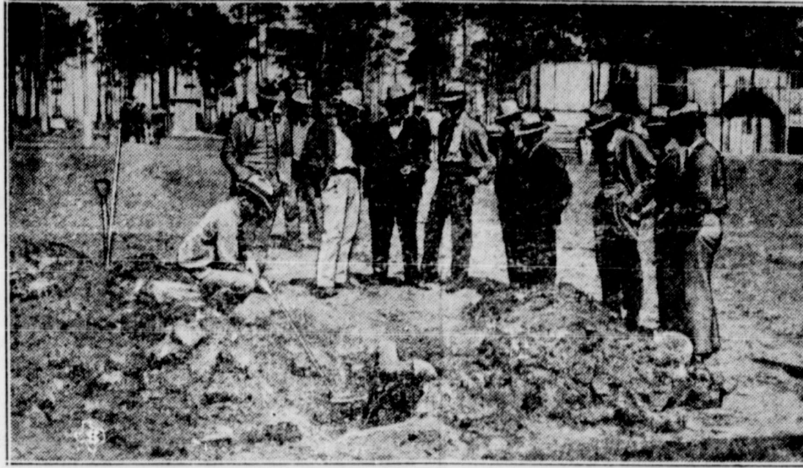
The Texas Railroad commission declared an open season on the lowly by-pass in the East Texas oil fields, and a number were captured in short order. A by-pass is a secret channel for oil, running oil off through a by-line. Sometimes the well owners place by-passes on their lines to slip the oil out of the field in defiance of proration laws. Sometimes thieves put by-passes on line and steal the oil. The above photo shows Lane Finley with a prod pole pointing to a by-pass near Glade-water. The big man in the center is Texas Ranger George H. Johnson.
