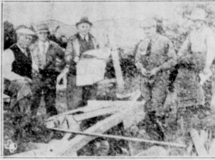
Here are the first views of construction work just begun atop Mount Locke, Davis Mountains of West Texas, on the Mount Locke Astronomical Observatory, which will be the second largest in the world. In the picture are several members of the construction company which will build the observatory, and at the right is Prof. G. Van Biesbroeck, astronomer of the Yerkes observatory, who will orientate the building with the stars. The observatory is being built by the University of Texas and the University of Chicago.
