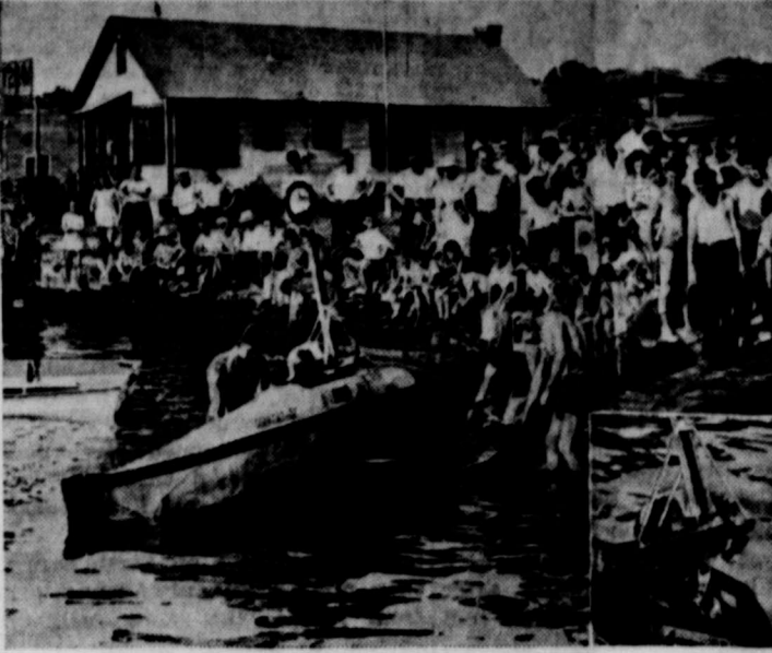
Barney Connett of Chicago, master and crew of an 11-foot submarine, previous to making a successful test dive in the salt water of the Hudson river in Yonkers, N. Y. Connett, in his homemade sub, has made approximately 400 dives, once crossing Lake Michigan under water from Chicago to Michigan City, Ind., a distance of 37 miles. The sub is powered by two sets of batteries and has all the usual submarine equipment.
