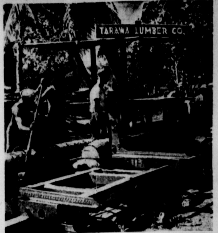
This sawmill was imported to Tarawa to aid in the reconstruction of the former Japanese base after the marines took it in the bloodiest battle of their history. The mill turns out lumber for tent frames, flooring and many other uses. The navy seabees and marine engineers have done a masterful job in improving this important Gilbert Island base.
