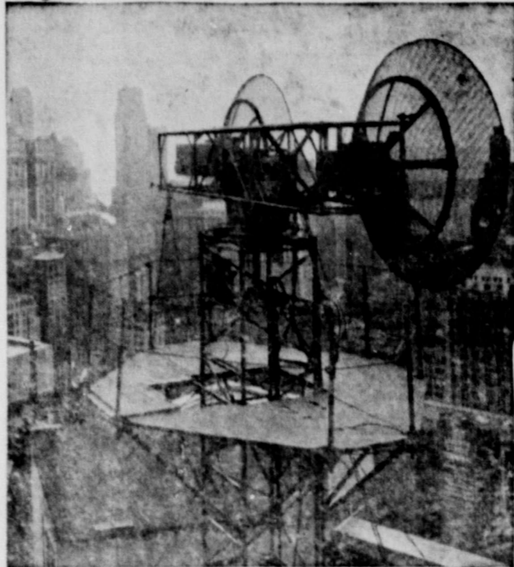
Shown atop the New York telephone building are the antennas used during demonstration of a secret army radar microwave relay system. The demonstration, conducted by Bell telephone laboratories, included a two-way voice transmission carried out successfully over links totaling 1,400 miles. It was announced as entirely practical and successful.
