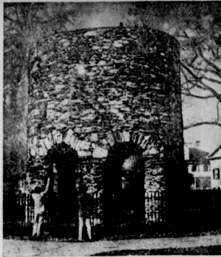
EARLIEST CHURCH—MAYBE... Excavation of this stone structure at Newport, R. I., may prove it to be the earliest Christian church in the western hemisphere. Research now is being undertaken by the Preservation Society of Newport to investigate the claim that it was built by Norsemen more than 100 years before the arrival of Columbus. Counter contention is that structure is simply an old windmill built in the 1600s by Benedict Arnold, then governor of Rhode Island.
