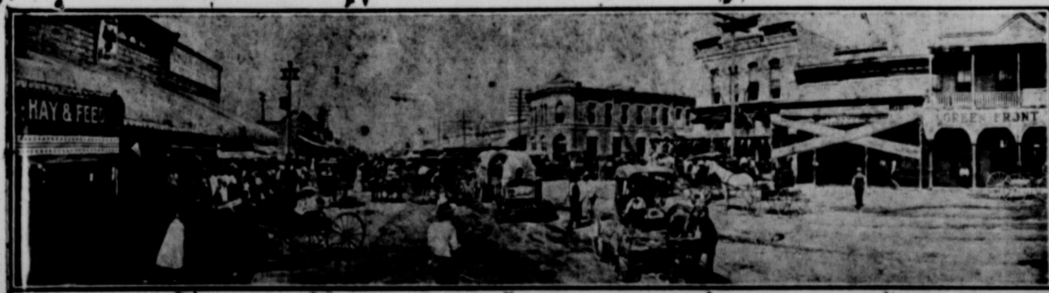
Ballinger pioneers gather for a June 29 celebration back in the early 1900s. Buggies, covered wagons and saddle horses provided the transportation, traffic rules were not a handicap to driving, paved streets were not dreamed of, and parking meters had not been invented. The wide-awake firm provided a hitching post at the curb, and red, white and blue bunting gave the town a "new look" for the gala program. Open saloons were in evidence along the main street.
