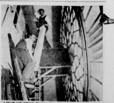
LIGHT UP BEN'S FACE-Behind one of the four faces London's famed Big Ben, workers Eric Lucas, top, and Harbour install one of the 56 fluorescent-type lighting fixtures. which will illuminate the massive clock for the first time and 1954. The fixtures are replacing the ordinary electric
