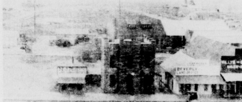
OLD FOARD COUNTY JAIL—The younger generation would not recognize this scene which was taken from atop the court house. It is a view to the south side of the square and shows the old Foard County jail before the present jail was constructed.
