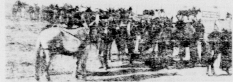
MULE POWER—C. H. McLellan of Wichita Falls, contractor for grade and drainage structures preparatory to paving U. S. 70 to the Wilbarger County line, first set up camp just east of Crowell. Portable food and housing facilities were provided, along with equipment for feeding and caring of his many mules.
