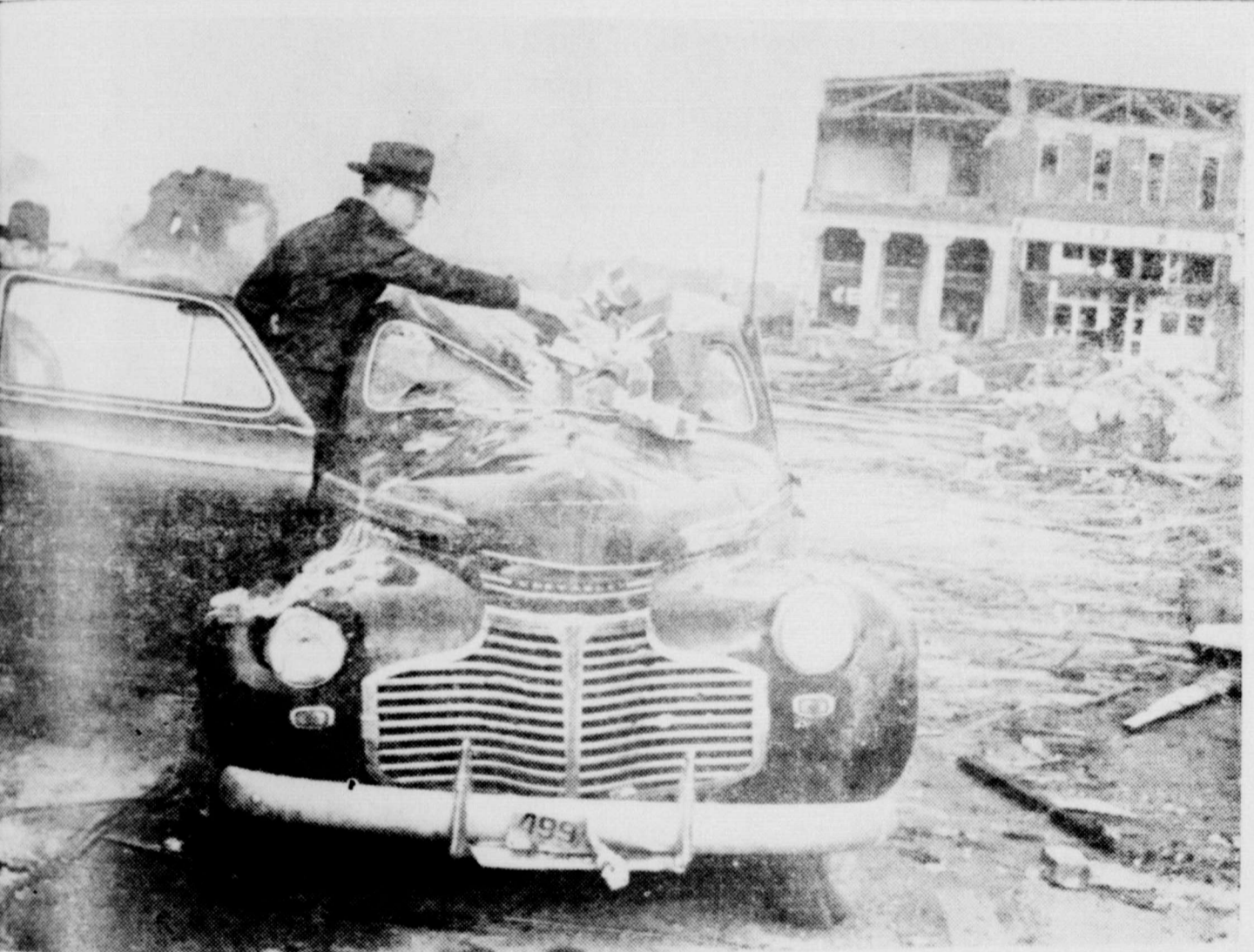
ALFRED EDDY INSPECTS CRUSHED CAR (ASCS Office in background)
