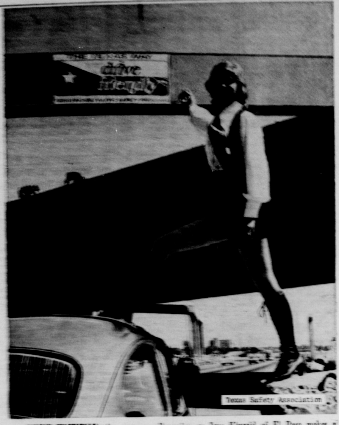
DRIVE FRIENDLY takes on a new dimension as Gene Kincaid of El Paso makes a pointed plea for Texans to heed the message of the world's heaviest billboard. Erected during a highway construction project on Interstate Highway 10 in El Paso, the 210,000 pound steel beam billboard is 45 feet above the ground. Using the beam for the Drive Friendly message was the brain-child of J. D. Abrams, President of the El Paso Traffic Safety Council, who says that driving friendly means not driving while under the influence of alcohol or drugs.
