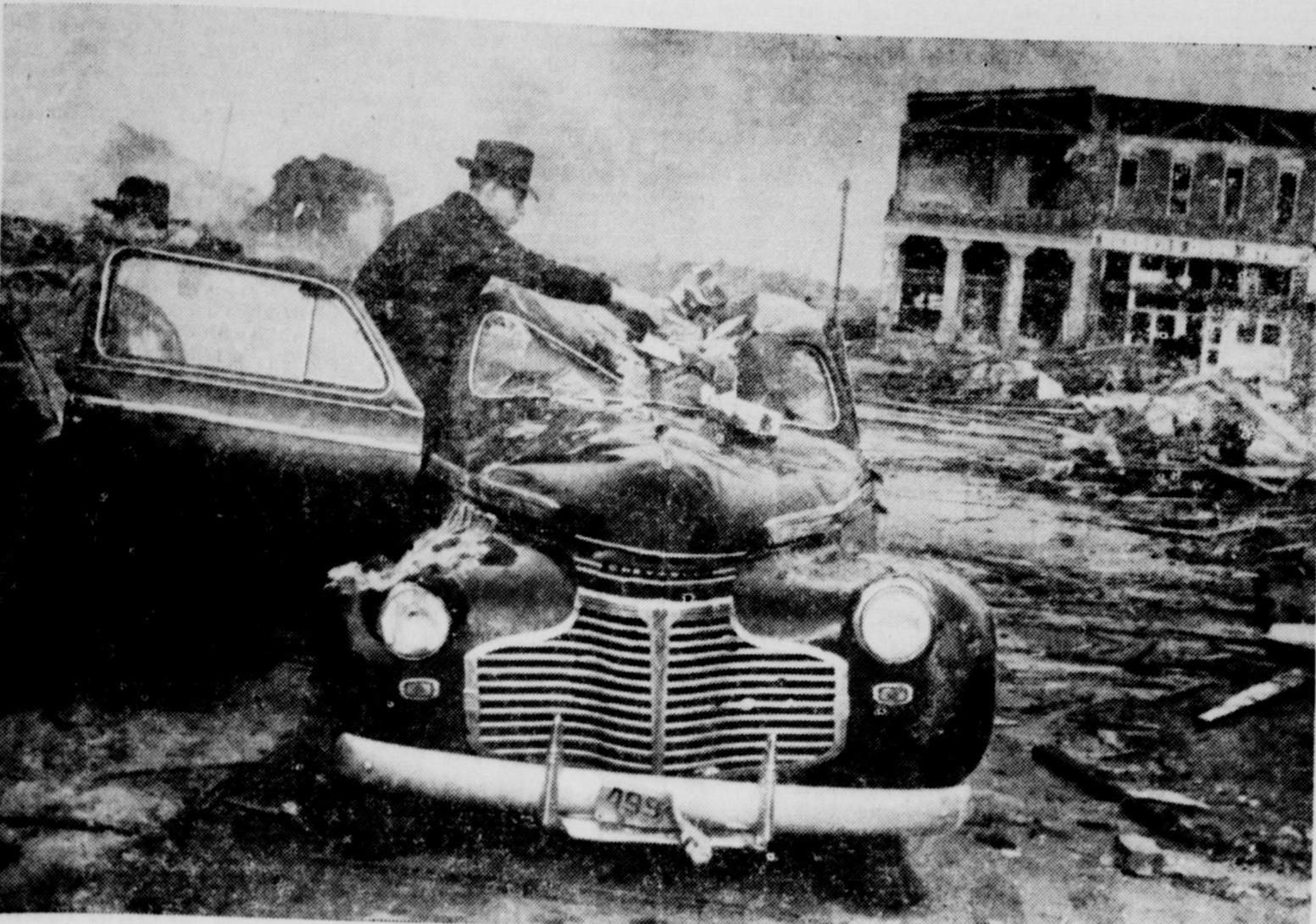
Alfred Eddy Removes Bricks from Battered Car
