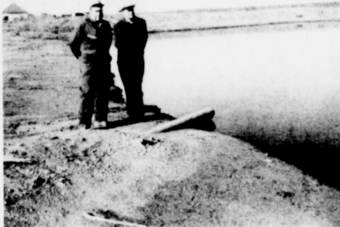
Pollution abatement holding pond on Borchardt farm.
