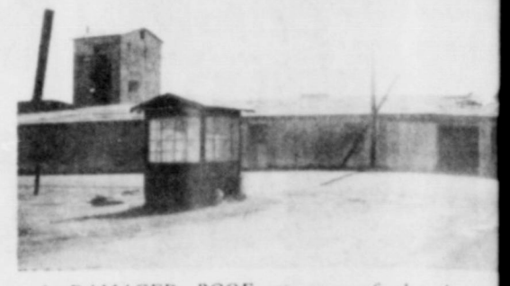
A DAMAGED ROOF at one of the three warehouses that were damaged by the storm.
