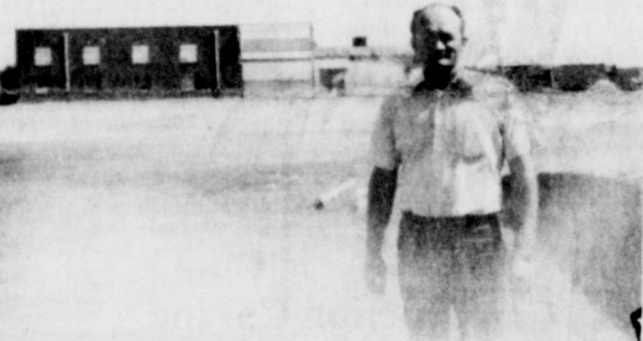
DALE READ, superintendent of O'Donnell schools, stands in front of the construction site for the new 4,000-plus square foot school building to be completed by the 1979-'80 school year.
