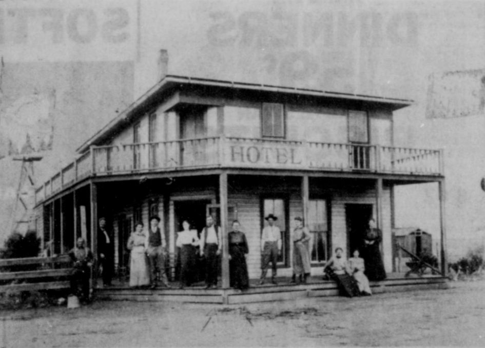
STOKES HOTEL in about 1904 or 1905 was located in the block now occupied by Lynn County Agriculture building and Fenton Insurance Agency. Mr. and Mrs. J.E. Stokes, owners are standing by corner post. (Photo given Tahoka Museum by "Buck" and Neva Barnes of Clovis, N.M.)
