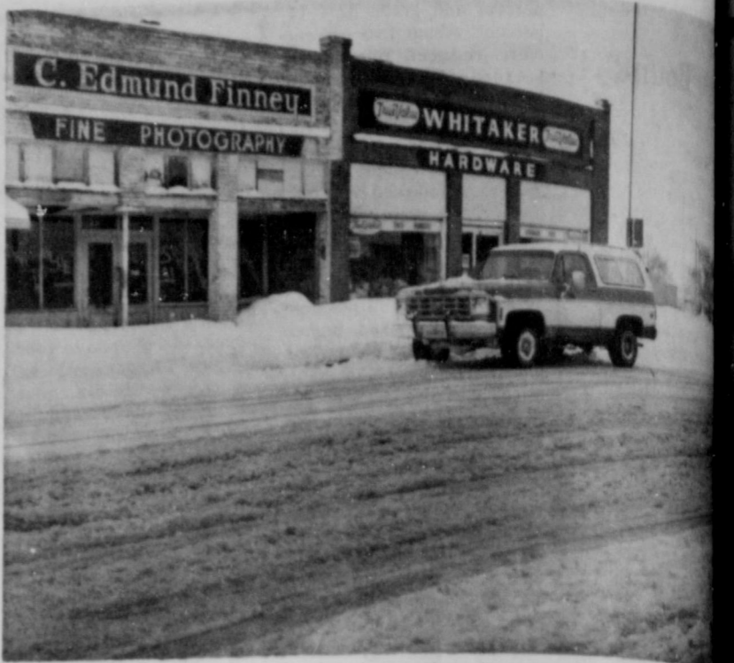
THAT DEEP--This Main St. photo shows how deep the snow last week drifted and how deep it is now. There was not much downtown activity last Wednesday. (LYNN COUNTY NEWS)
