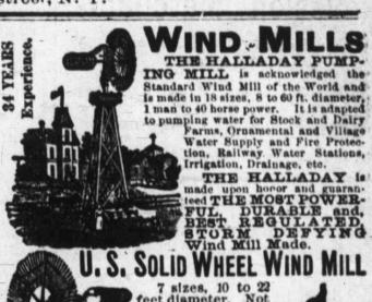
feet diameter. Not cheaply made but heavy and strong in construction. These Mills are taking the lead of all Solid Wheels on the market, and are guaranteed the Best of their class.
