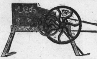
Crushing corn with shuck on or off, wet or dry, hard or soft, at the rate of 100 bushels per hour with two-horse power. Circulars
