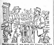
BRICKLAYER-If you want this Cistern to hold ust 200 barrels, how are we to determine its septh and diameter, and also the number of brick is will require to wall it up. CONTRACTOR-I see by R's C: (p. 62) that it must be 9½ feet in diameter, and 12 feet deep; and it will take 1,560 brick, if laid on edge or 3,000 if laid flat.
