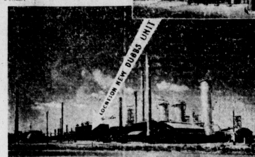
This installation will increase the output of HIGHER OCTANE GASOLINE by 175,000 gallons per day and will give the refinery sufficient capacity to completely process into gasoline and fuel oil 14,000 barrels of crude per day, and by manufacturing various grades of Diesel and furnace oil will give a flexibility of 17,000 barrels of crude oil per day.
