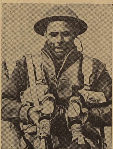
An Australian soldier examines two anti-tank bombs, taken from Italians at Bardia, Libya. The bombs are made of gasoline-filled bottles attached to hand grenades.
