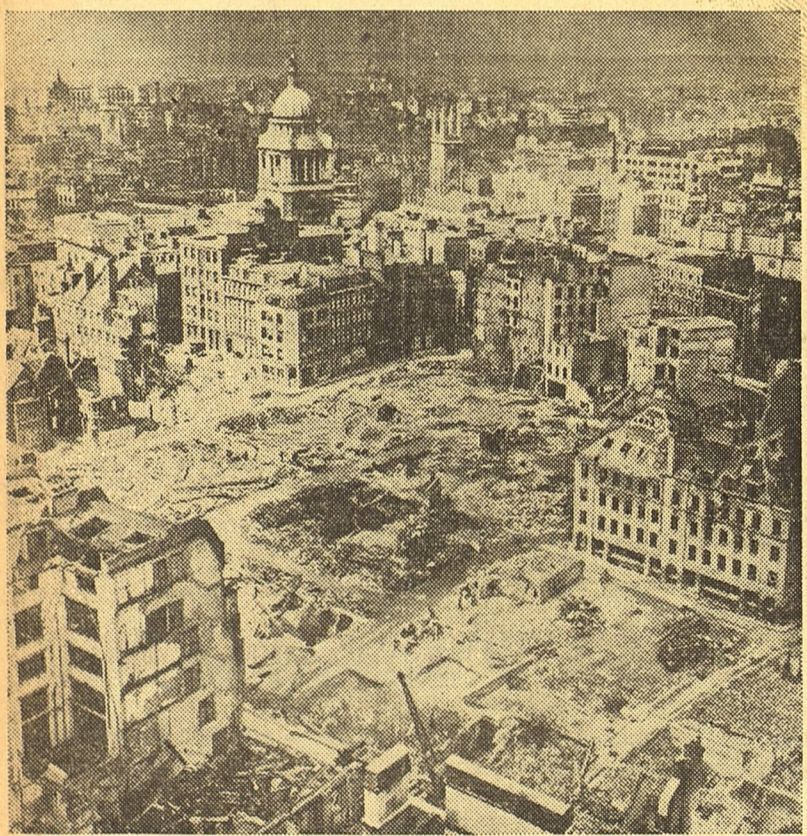
This photograph, just released by the British censor, shows some of the devastated sections in the center of London after air raid clearance work. An entire block of demolished buildings has been completely removed, leaving nothing but vacant lots, as shown in the picture.
