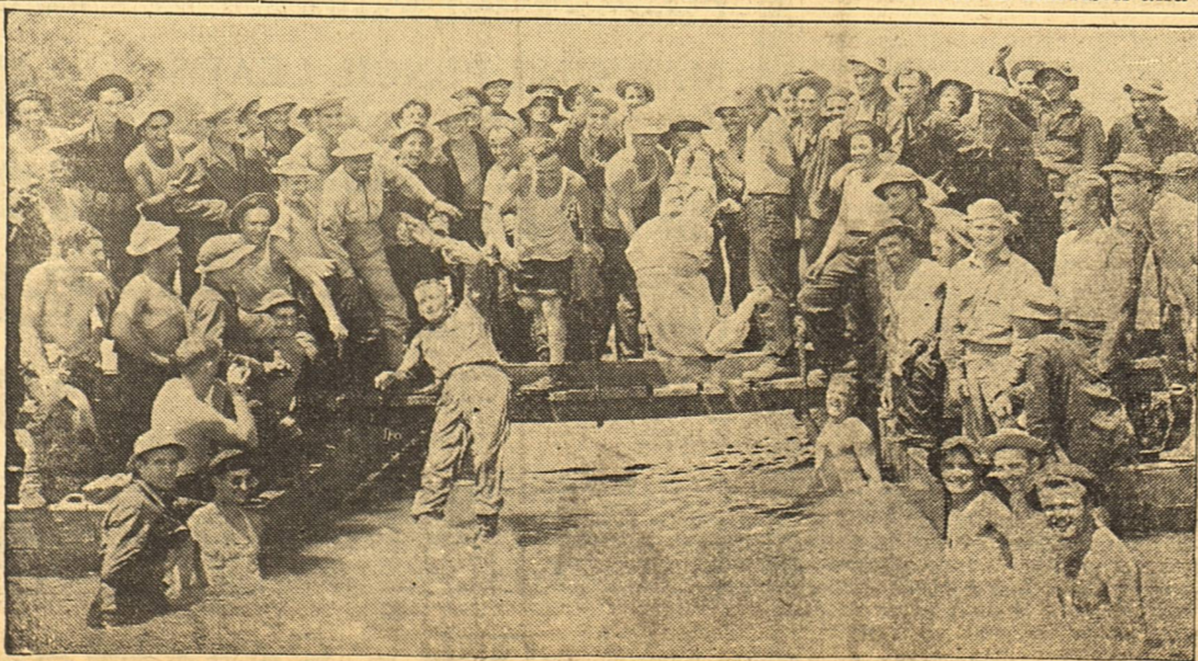
Members of the 108th combat engineers of Chicago, toss their commander, Col. Karl Hobart (left) and Lt. Phil Clementz (right) into Red River after completing a 658-foot pontoon bridge in less than a half a day. Starting at 6:30 A. M. the Colonel and Lieutenant had told the men they could throw them in the river if they finished the job before noon. They did. The bridge building was part of the maneuvers being carried out in Arkansas.
