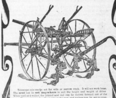
ter-balance the weight of light or heavy gangs. The spreader is adjustable from the seat by a haad latch. The hitch is low but with ample clearance. Wheels are 44 inches high, and have dust-proof removable boxes, permitting the use of hard oil. The Victors are "top-notchers" in every way.
