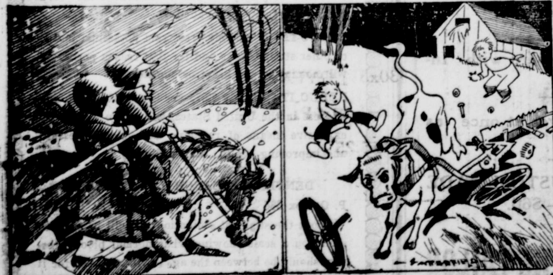
3. In winter Herbert and his cousin rode horseback to school two miles away. 4. The future engineer constructed a mowing machine out of an old cross-cut saw, using a heater for power.
