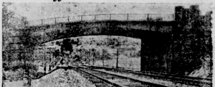
St. Pleasant Bridge, selected as one of the most beautiful short-span bridges in the world, is a splendid example of the steel overpass. It crosses the roadway over a formerly highly dangerous railroad crossing at Mt. Pleasant, New York.
