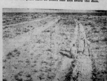
Contour ridges totaling 1,700 miles have been built on the McElroy ranch in Crane and Upton counties. The ridges are designed to hold the rain where it falls and to prevent rapid
