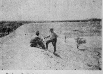
Tank on the D. S. Pumphrey ranch near Mercury, McCulloch county. The dam is made of 6,490 cubic yards of dirt and the tank will hold 36 feet of water, enough to serve cattle through a series of dry years.
