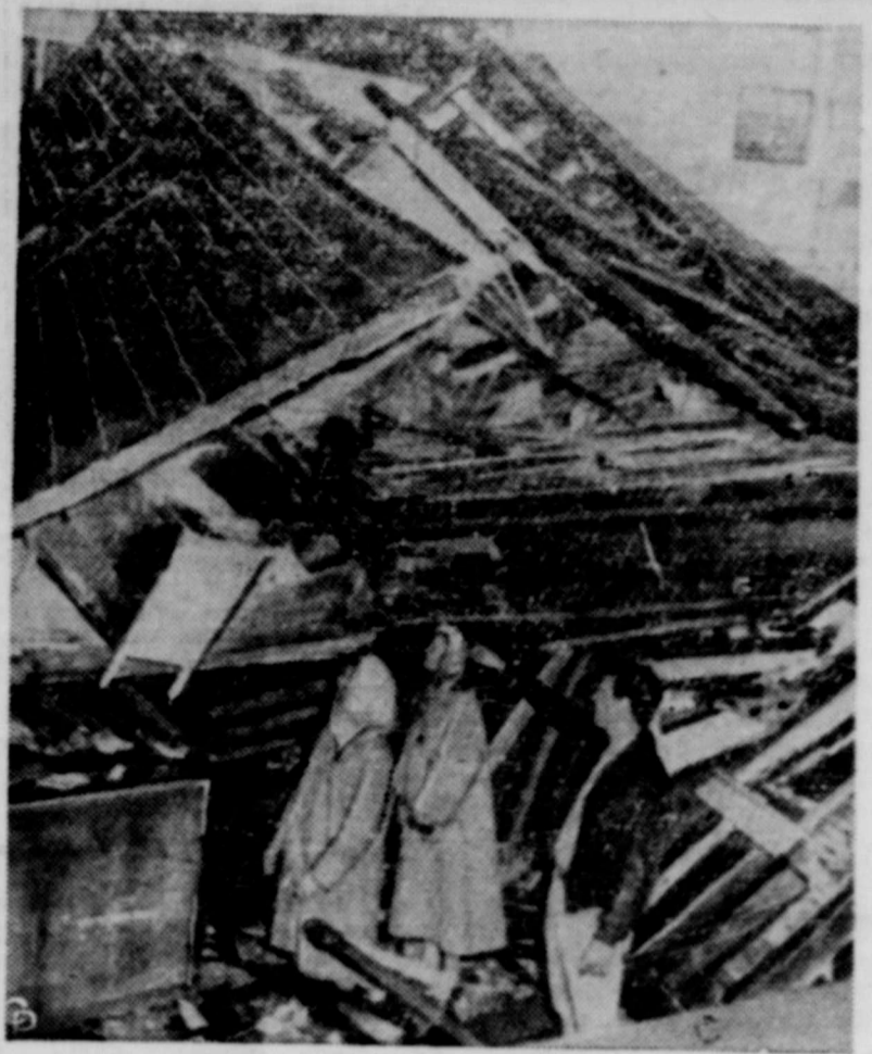
SIXTY-FIVE-MILE-AN-HOUR gale winds, whipping through the San Francisco Bay area, leave a home in ruins. Looking at the wreckage are Mr. and Mrs. Edward Campbell and his sister, Patricia. Trees were blown down, roofs were torn off and power lines disrupted.
