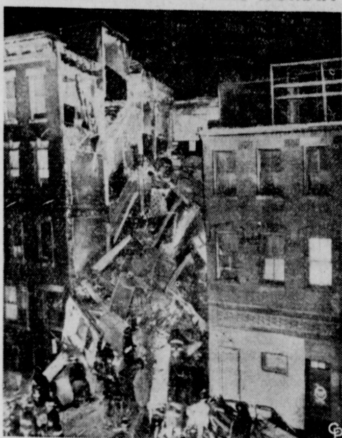
RESCUE WORKERS and firemen probe the ruins of a collapsed four-story, 150-year-old tenement in Boston. Later, the body of Mrs. Susan Johnson, 58, a cripple, was found wedged under a concrete slab. Several persons were injured. Officials said disintegrated billings caused the structure to collapse. (International Soundphoto)
