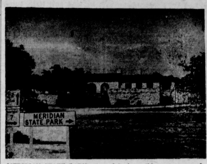
MERIDIAN STATE PARK returned to favor this year as one of Texas' popular fishing resorts. Water began flowing over the spillway of its dam on May 2, 1957 for the first time since May of 1951. During the dry years the lake level had dropped 21 feet. Weeds and rough fish were removed during the drouth and the lake restocked by the Game and Fish Commission.—Photo by Roger Parker.
