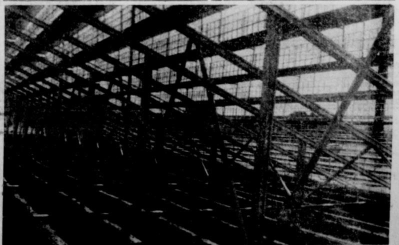
STEEL FRAMEWORK—This picture shows construction of the new bleachers from the underside, looking from the northwest toward the southeast. As this picture would indicate, a large amount of surplus steel rails and steel landing mats was utilized in this construction job.
