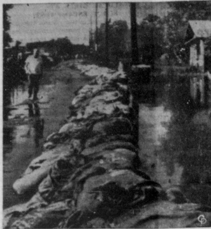
RANKS OF THE WABASH SPREAD —Water seeps through a sandbag levee in Terre Haute, Ind., as the Wabash River continues to overflow its banks. More than 5,000 persons waged an around-the-clock battle to keep the rising waters back. Indiana's Gov. Harold Handley has declared an emergency.
