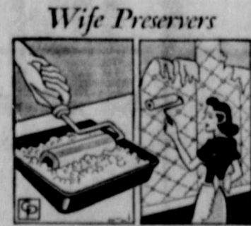
A point roller, covered with warm soap or detergent suds, can be used to remove wallpaper.
