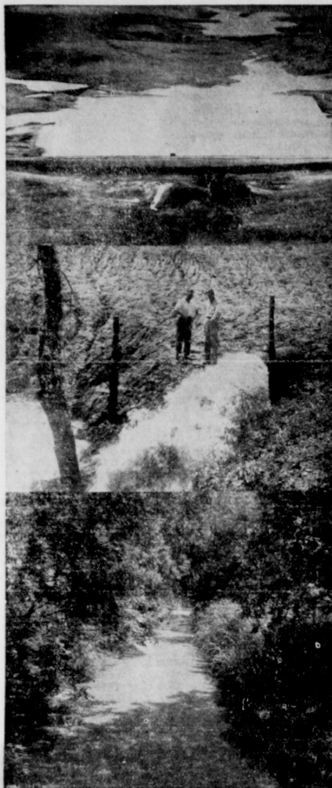
TOP:—Flood water held behind retarding structure. CENTER:—Discharge from drawdown tube. BOTTOM:—Stream is about one-third full but is not overflowing.
