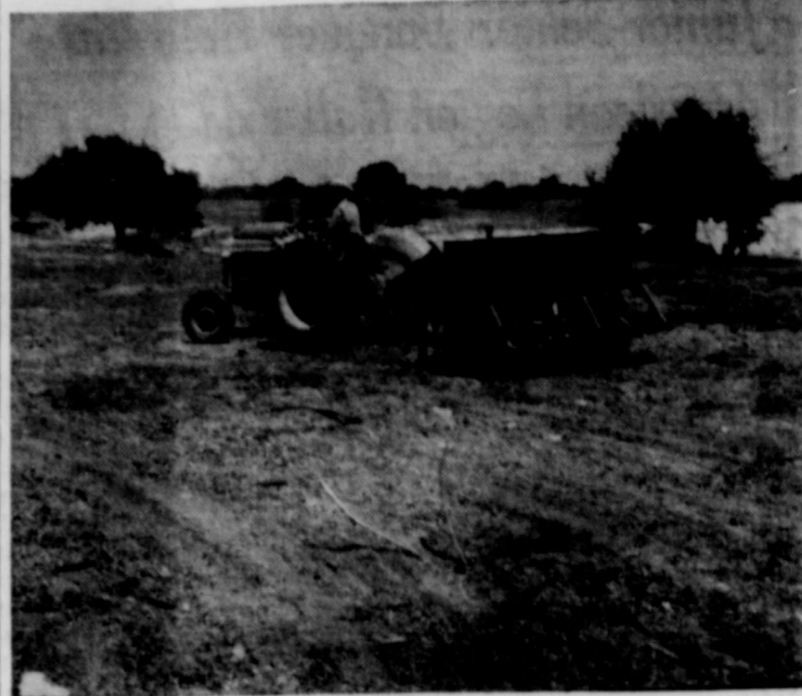
SEEDING GRASS —Barney Welch of Mullin used the district drill to seed Side Oats Grama and Green Sprangle Top following Mesquite brush control. The grass drill shown has depth band gauges and double disc openers, important in proper placement of grass seed. About 250 acres of grass were seeded with this equipment this spring. —(SCS Photo)
