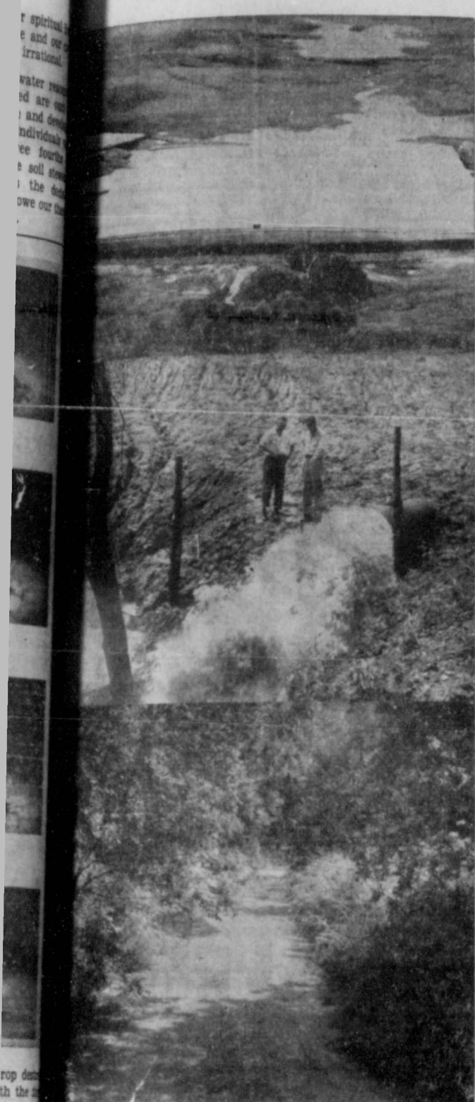
Flood water held behind retarding structure. Discharge from drawdown tube. Stream is about one-third full but is not overflowing.
