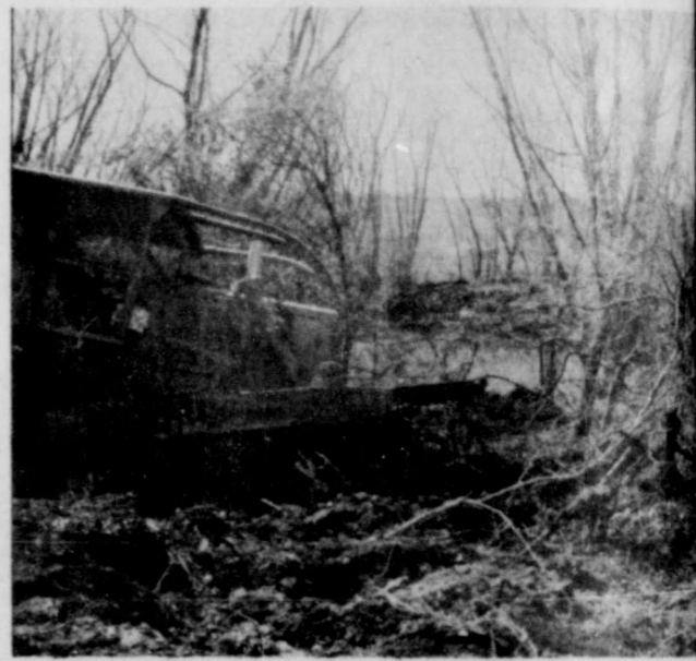
Contractor tree dozes brush on the Glynn Collier Ranch north-east of Goldthwaite. Collier will follow-up with highway tandem and farm tandem prior to sprigging to coastal bermudagrass. SCS Photo
