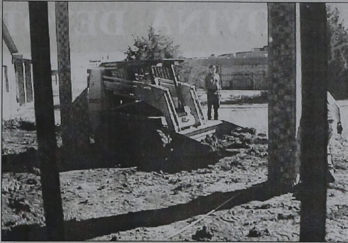
WORKMEN ARE shown tearing out the concrete patio at Friona Heritage Estates. The original patio was not properly graded and caused water to drain into the Heritage Estates dining area. New concrete was poured to drain away from the facility. ron carr photo
