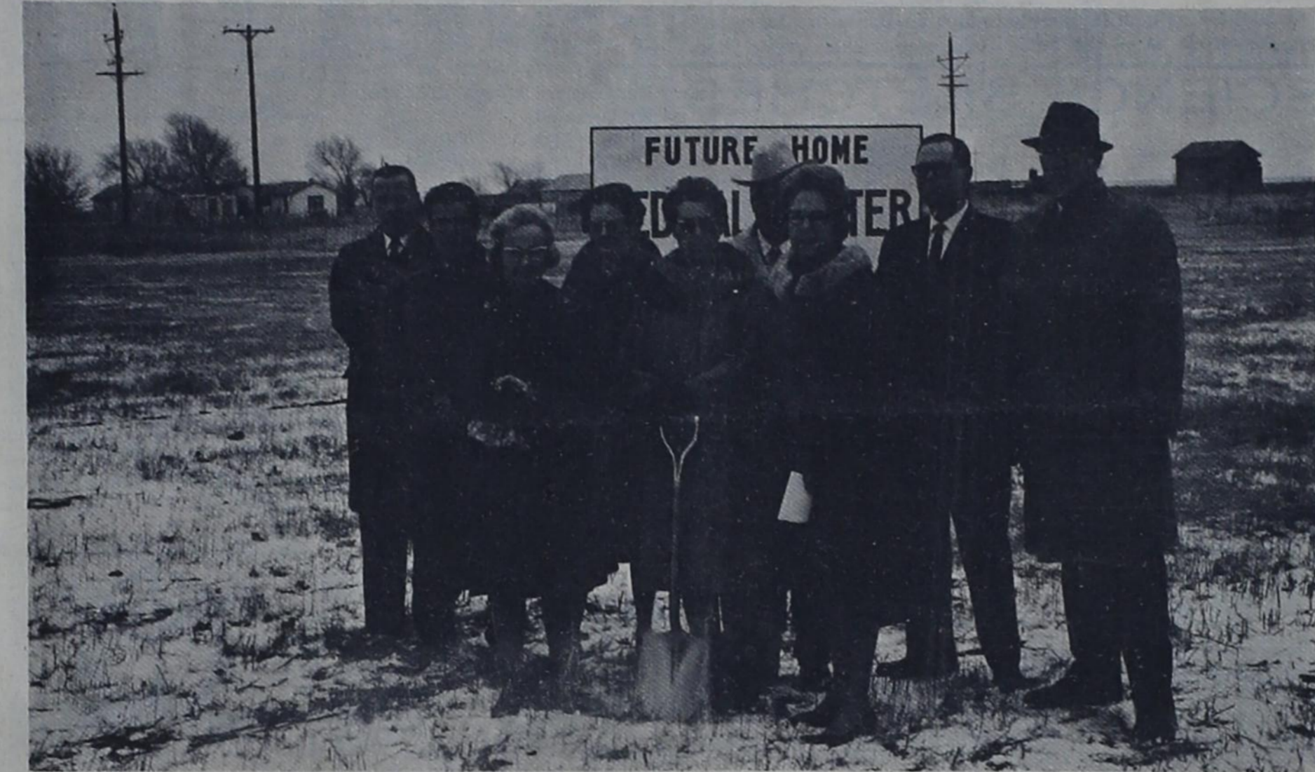
GROUND BREAKING -- Ground was broken by a golden shovel Sunday afternoon at the site of the new Bovina medical clinic near Highway 1731. Among those attending the event were, left to right, J. E. Sherrill, contractor; Fred Langer, a member of the Joe Langer family which donated the land; Mrs. Jesse Walling, community project chairman of Bovina Woman's Study Club; Mrs.
