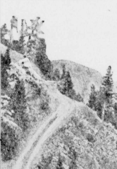
Improved Road in Oregon.
