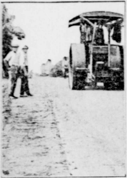
Building Federal-Aid Roads—the Kind That Stand the Wear.
