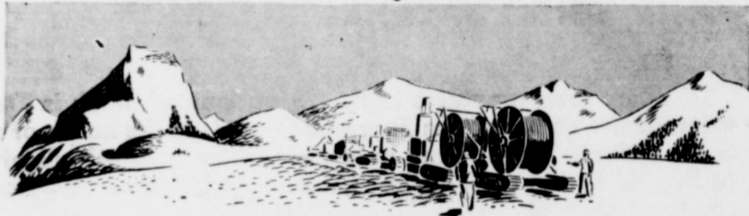
Giant plow train trenches cable over mountains and across deserts
