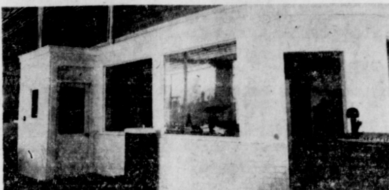
Here is shown the modernistic office in Linkenhoger's new store. —the heart of the business, and located right in the center of the building.
