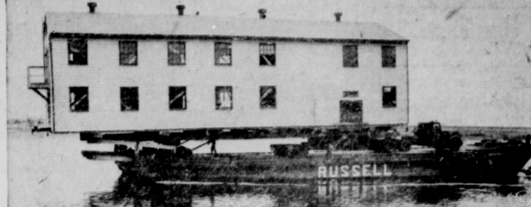
Barracks, formerly used to house atomic workers at Hanford, Wash., are being moved to Richland, 24 miles away, where a new city is springing up as the Richland Engineer Works is expanded. This building, going by truck, crosses a waterway by barge. The barracks city will eventually provide homes for 16,000 persons at Richland.
